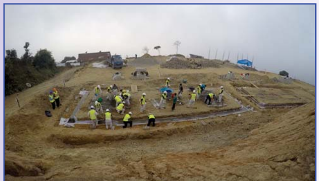
Ground enabling work at Jiri
