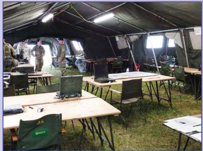
The VE Gp HQ build in progress
