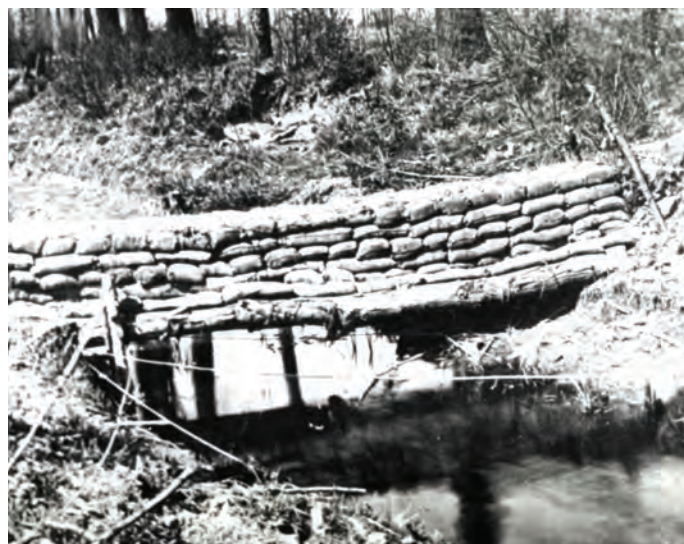
Buried Cable Crossing a Stream. This image illustrates the labour intensive protection required for fixed line cables. Image courtesy of the Royal Signals Museum.
